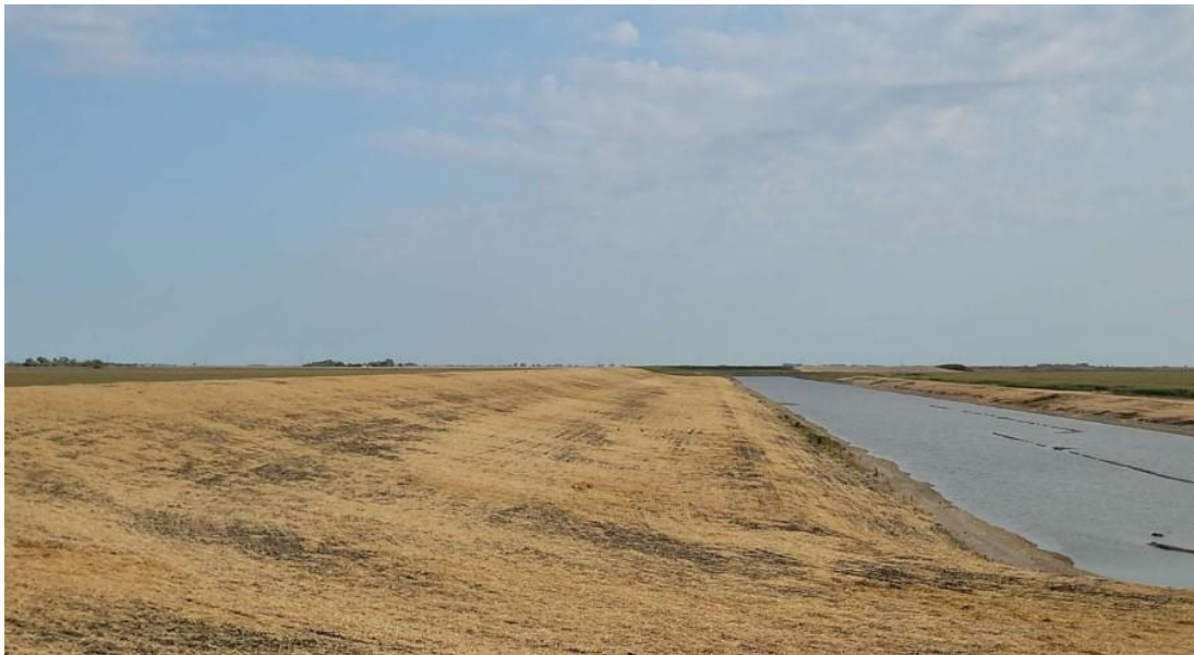
Reddpath Impoundment Construction
